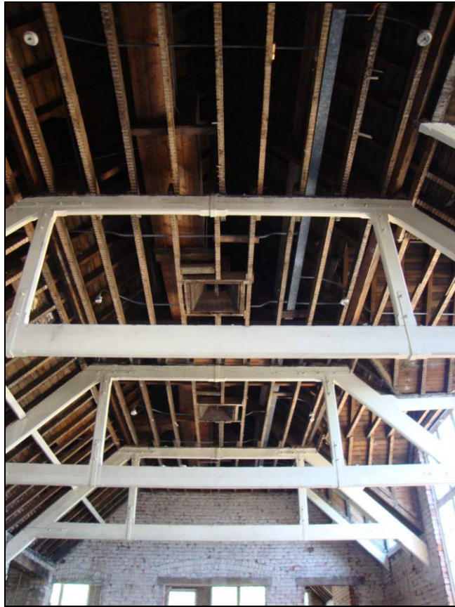
Figure 43: Roof detail of Room 4.
