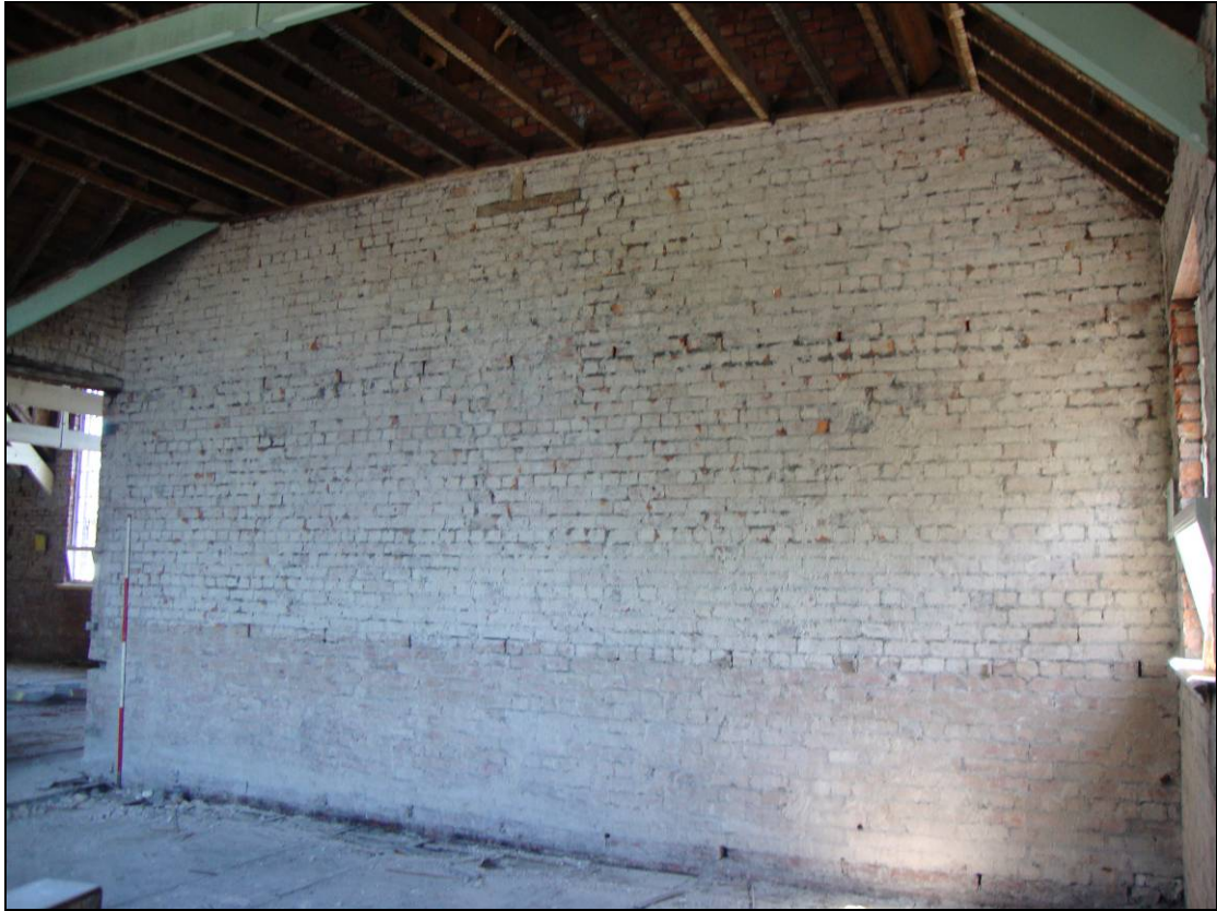
Figure 62: North elevation of Room 9, looking north. Scale = 2m
