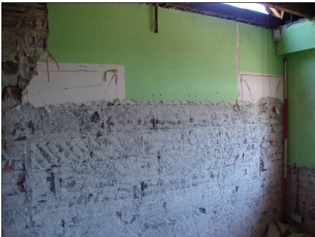
Figure 33: West elevation of Room 2, looking north west. Scale = 2m
