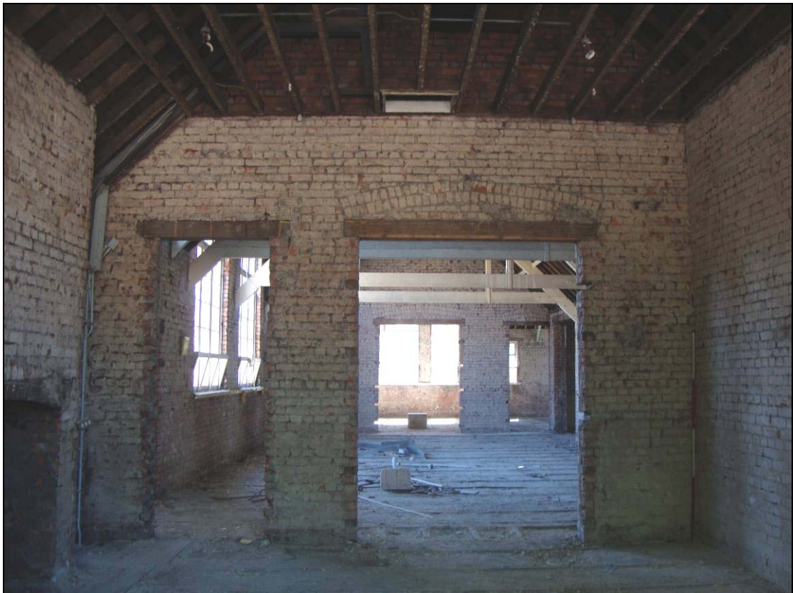
Figure 45: East elevation of Room 5, looking east. Scale = 2m
