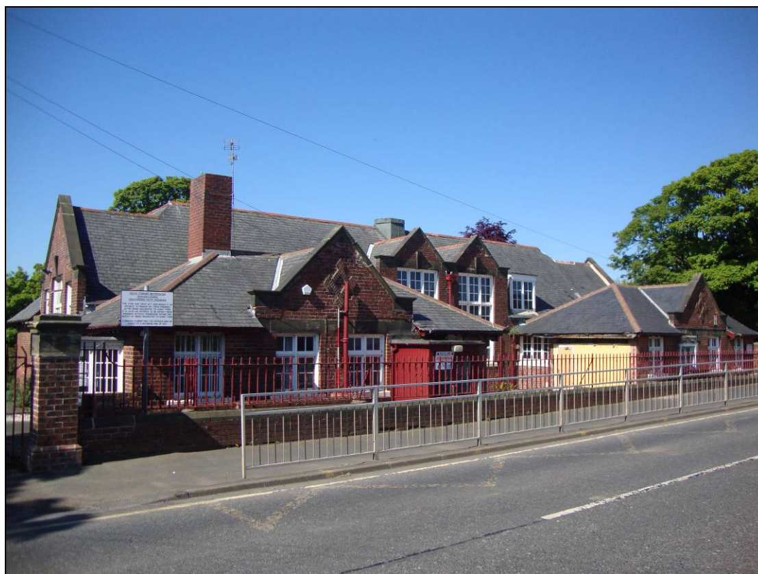
Figure 21: North facing elevation, looking south west. Scale = 2m
