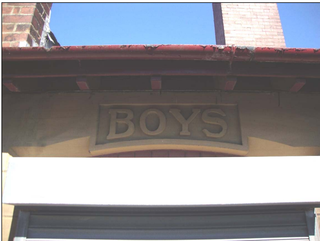
Figure 20: 'Boys' inscription above the blocked doorway into the boys' cloakroom.
