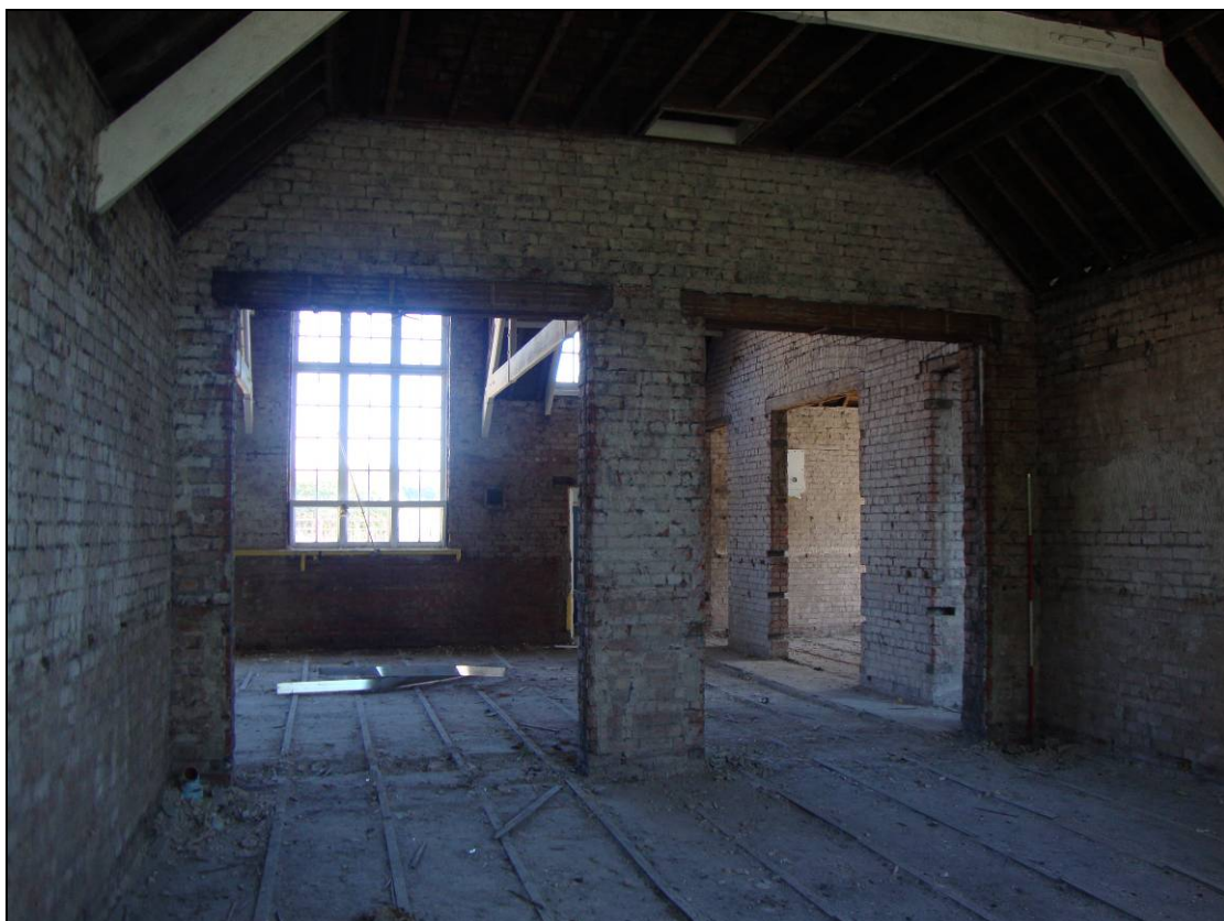
Figure 55: North elevation of Room 8, looking north. Scale = 2m
