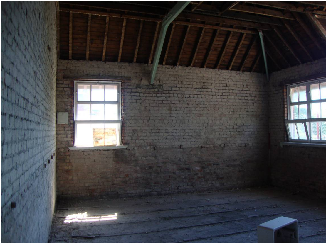
Figure 59: East elevation of Room 9, looking east. Scale = 2m
