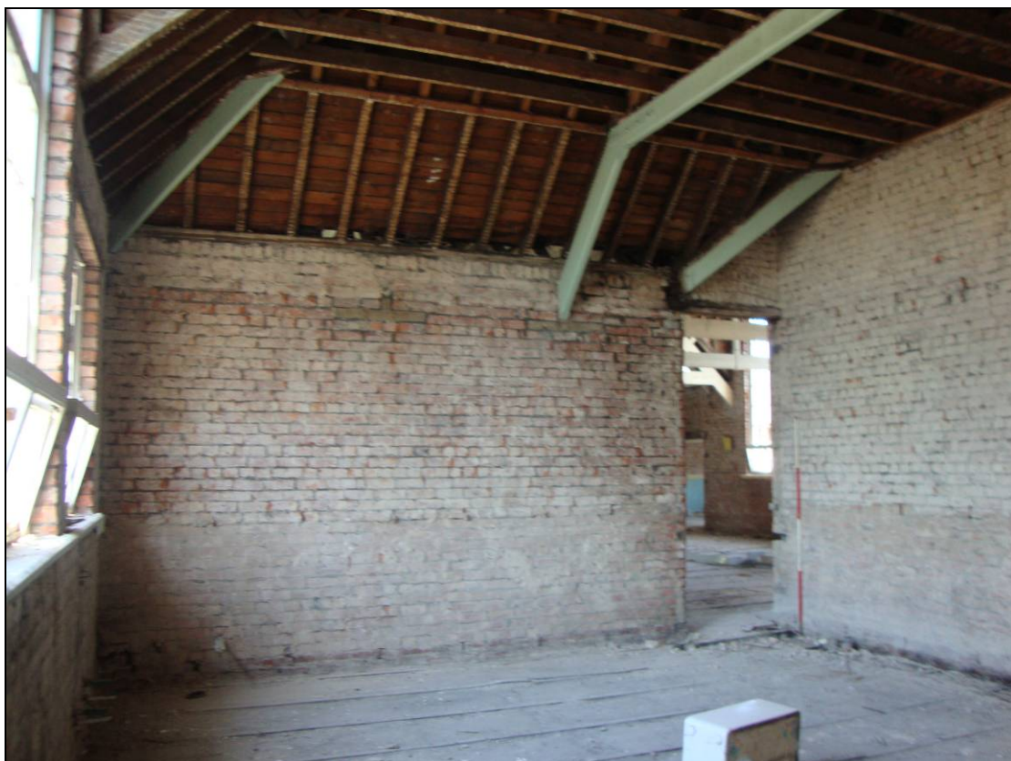
Figure 61: West elevation of Room 9, looking west. Scale = 2m
