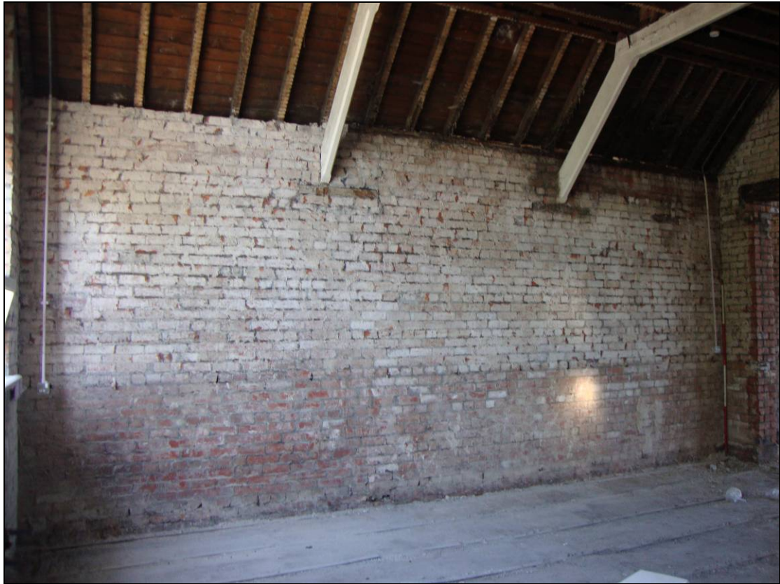
Figure 51: West elevation of Room 7, looking west. Scale = 2m
