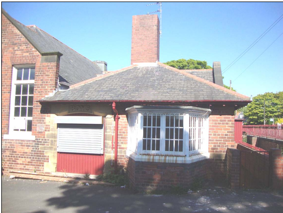
Figure 19: Northern extent of east facing elevation, looking west. Scale = 2m
