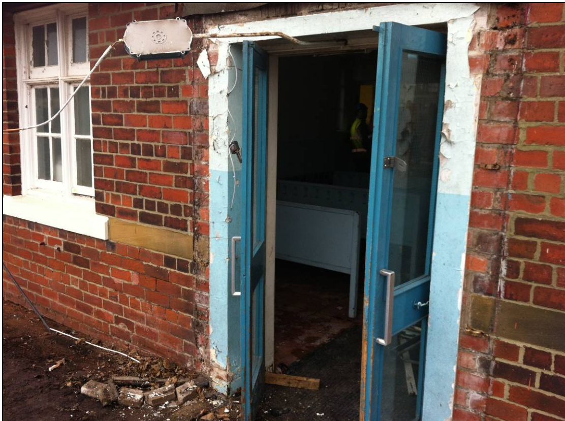
Figure 7: The western front porch, after demolition. Note coat hooks inside.
