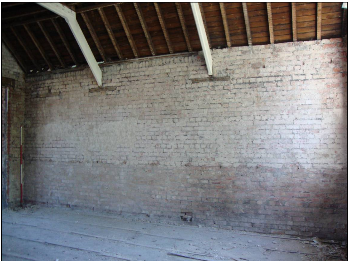
Figure 58: East elevation of Room 8, looking east. Scale = 2m
