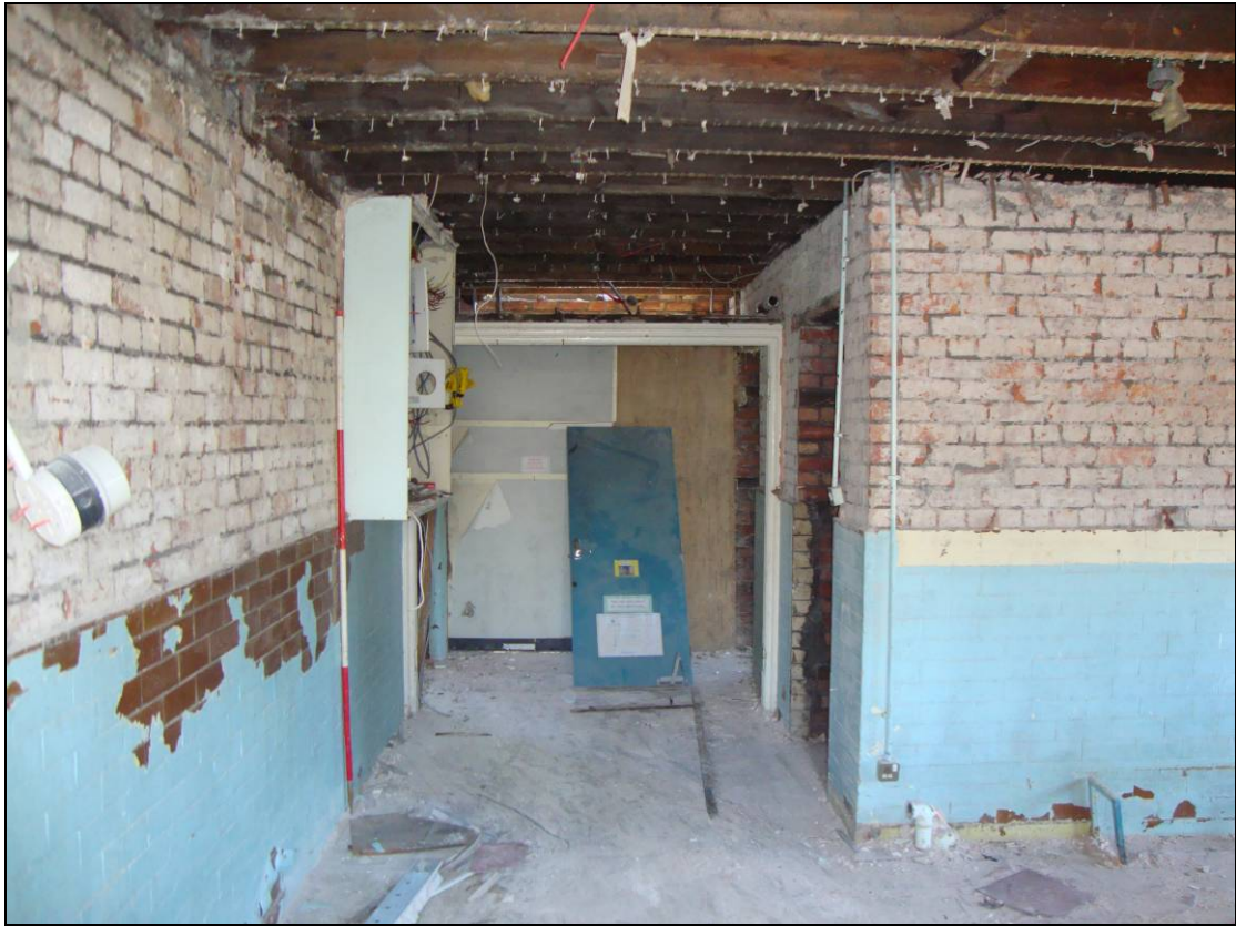
Figure 32: West elevation of Room 1, looking west. Scale = 2m
