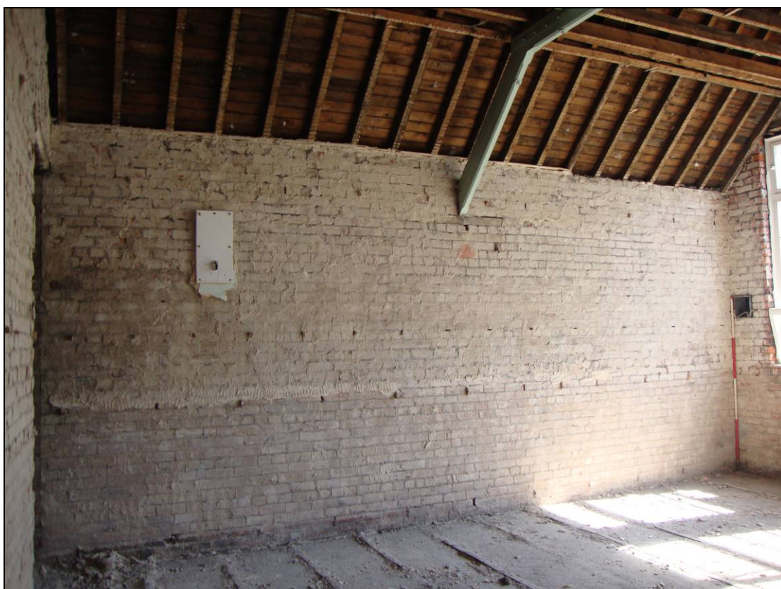
Figure 64: North elevation of Room 10, looking north. Scale = 2m
