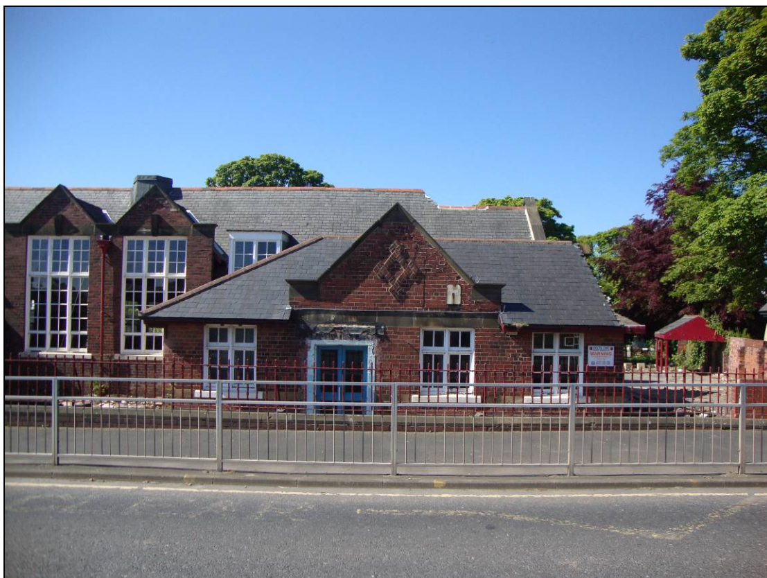
Figure 24: Western extent of the north facing elevation, looking south.
