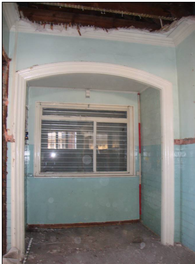
Figure 70: Southern extent of east elevation of Room 11, looking east. Scale = 2m
