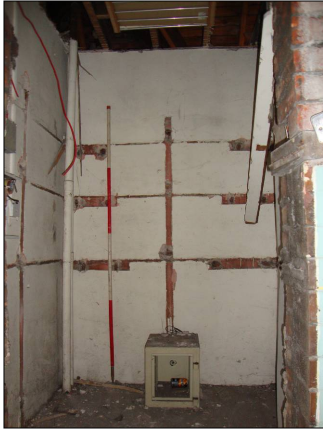
Figure 71: Room 12, looking north. Scale = 2m
