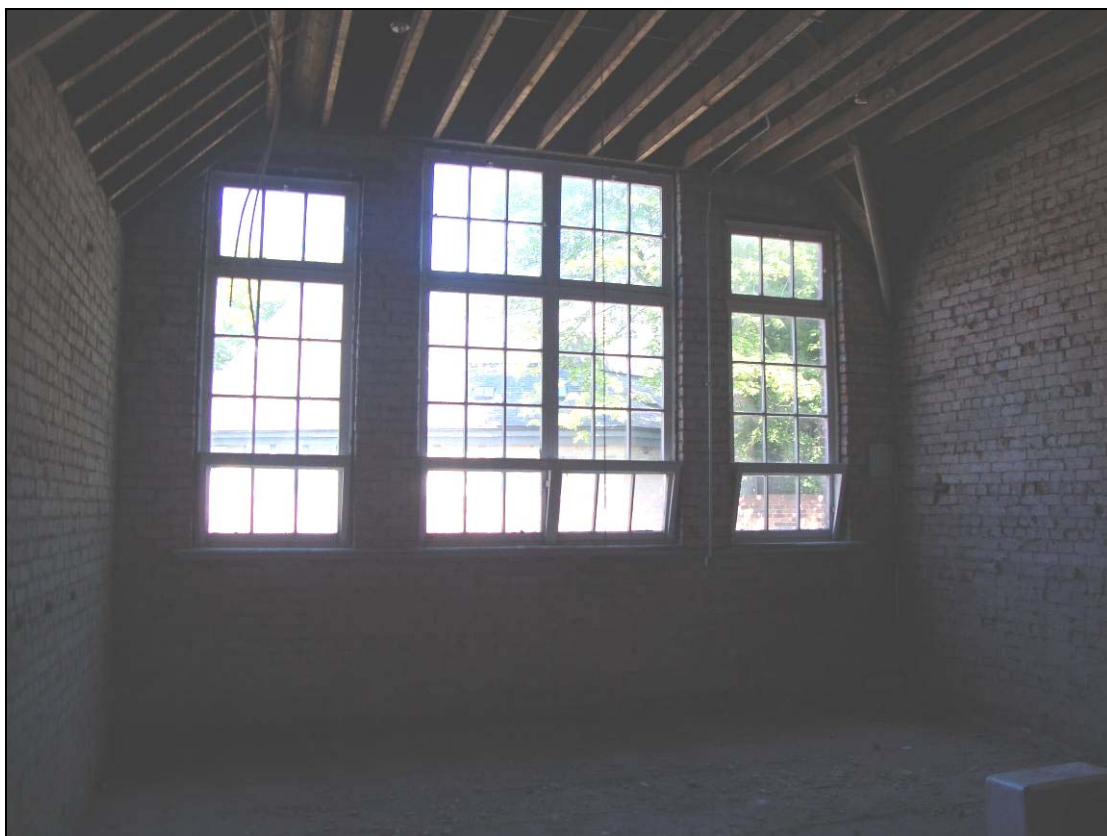
Figure 50: West elevation of Room 6, looking west. Scale = 2m
