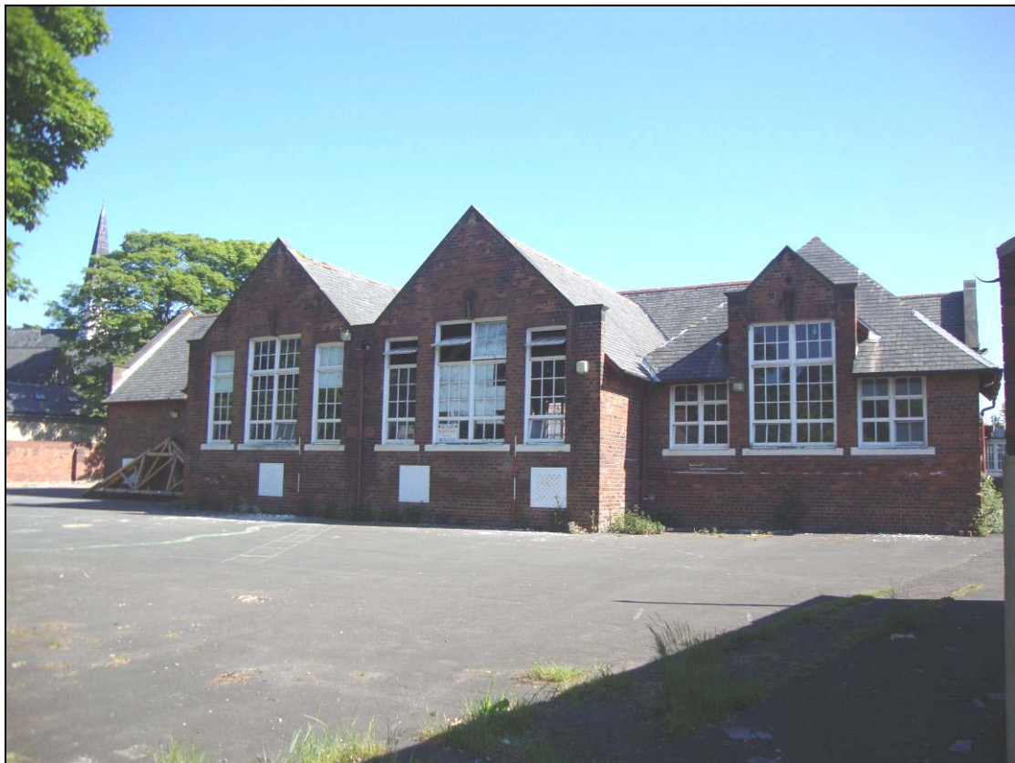
Figure 15: South facing elevation, looking north. Scale = 2m
