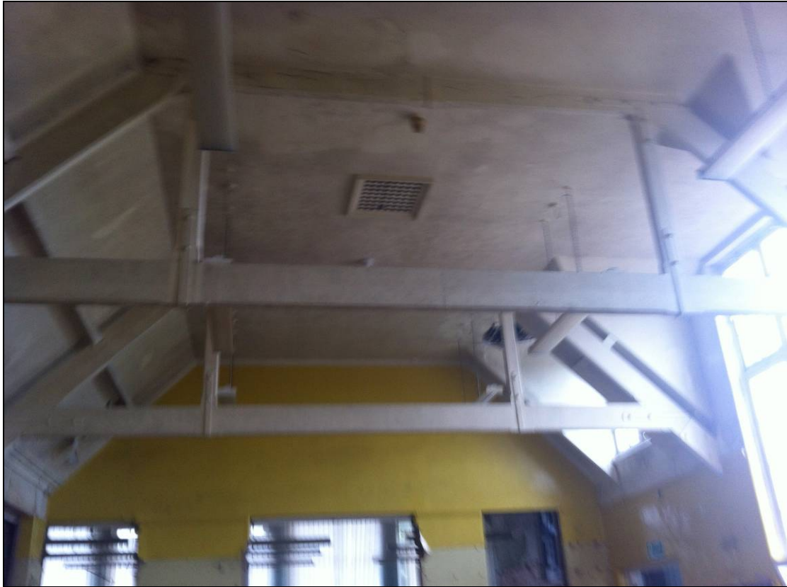
Figure 6: Detail of the ceiling in the main assembly hall, looking west
