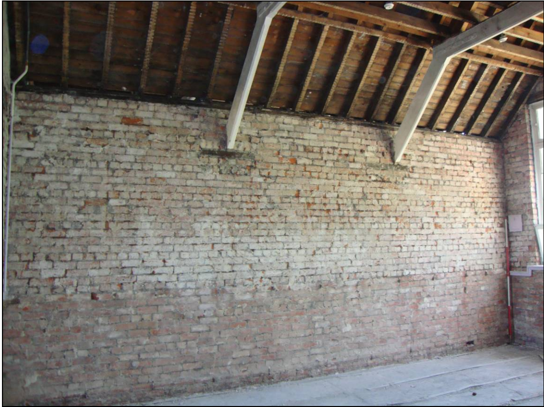
Figure 54: East elevation of Room 7, looking east. Scale = 2m
