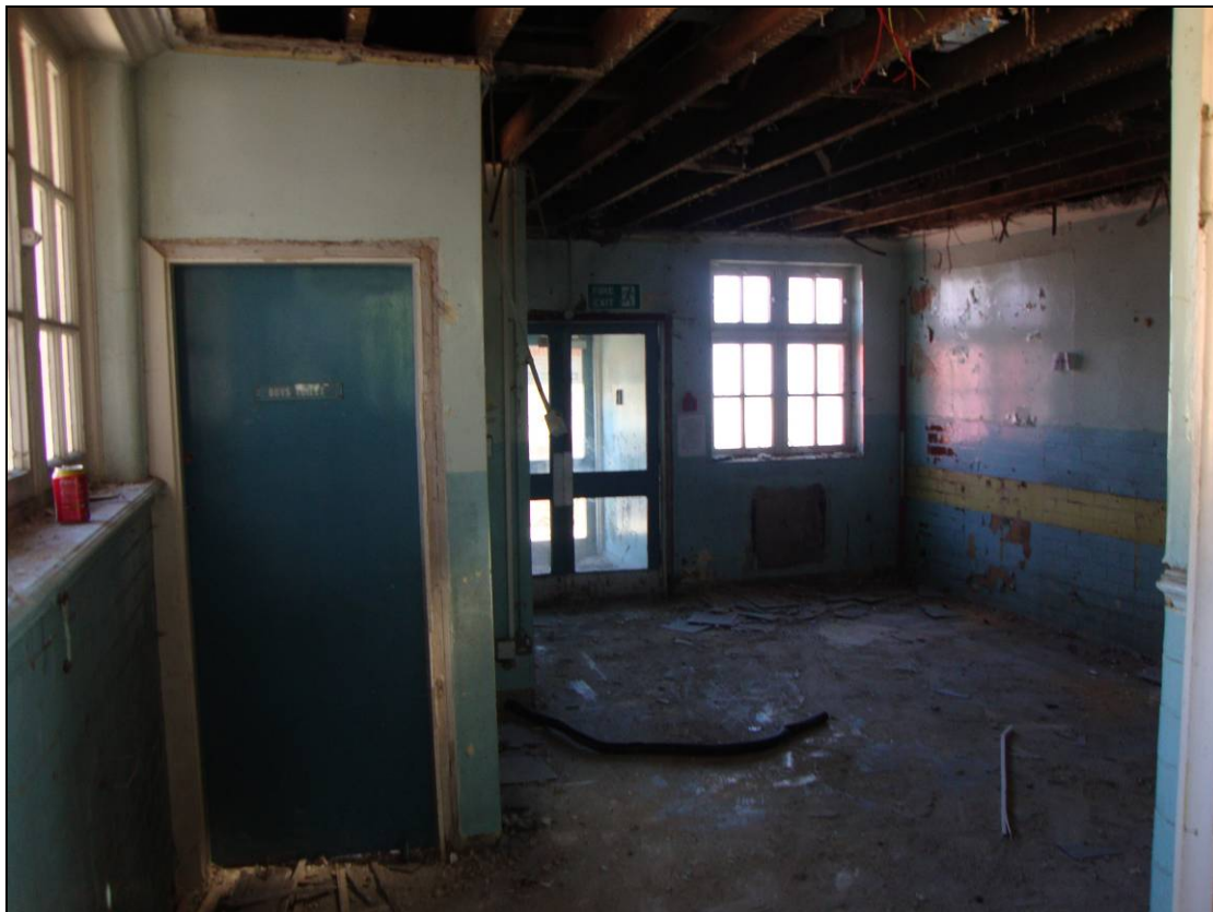
Figure 67: North elevation of Room 11, looking north. Scale = 2m
