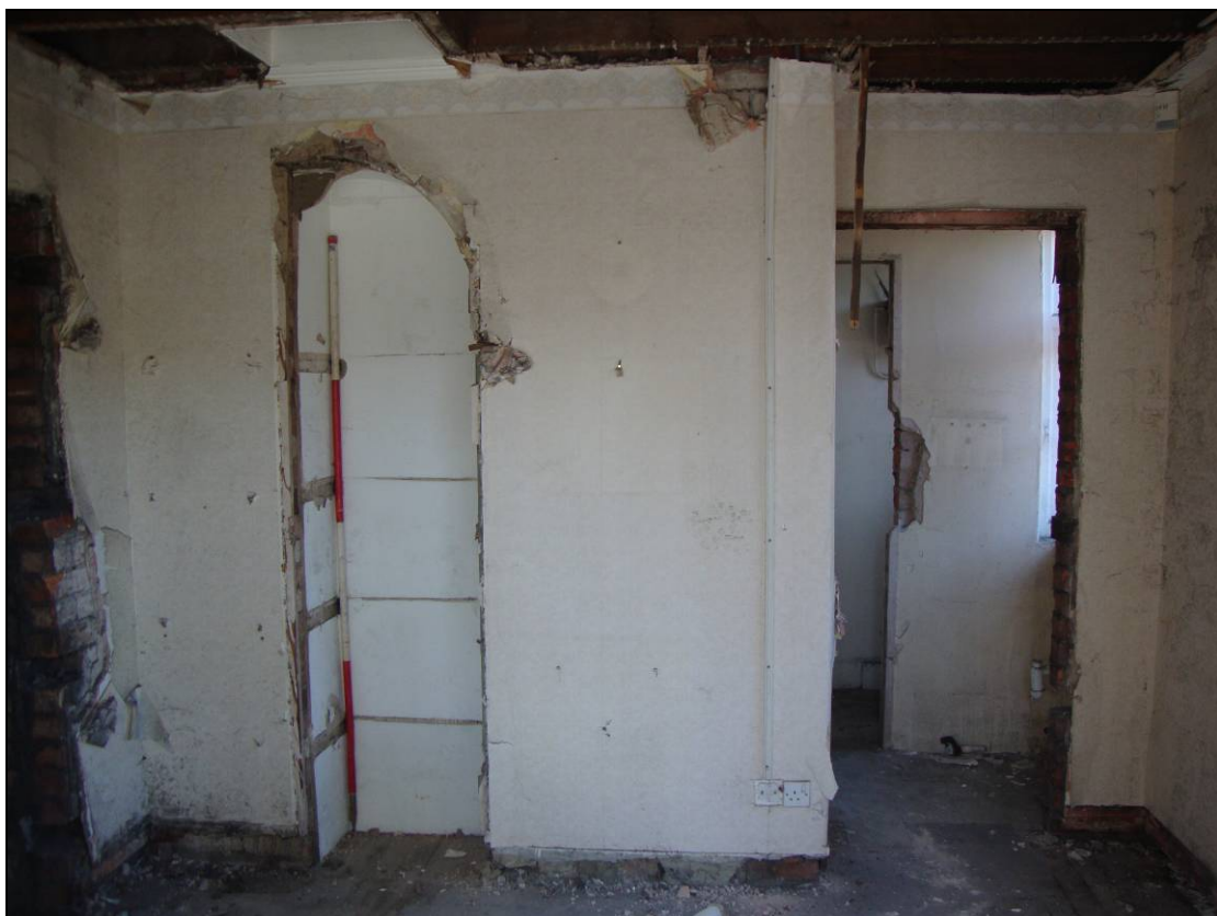
Figure 72: West elevation of Room 13, looking west. Scale = 2m
