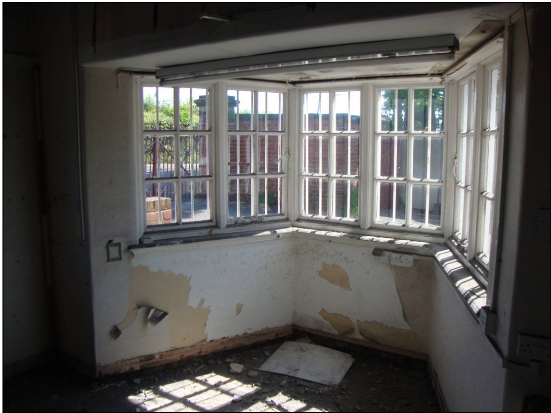
Figure 74: East elevation of Room 13, showing detail of bay window, looking east. Scale = 2m
