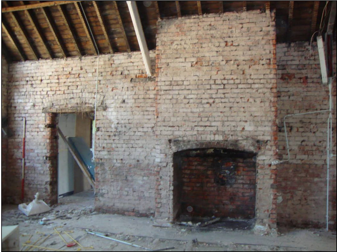
Figure 44: North elevation of Room 5, looking north. Scale = 2m
