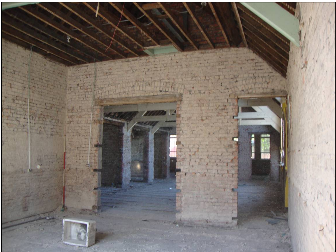
Figure 66: West elevation of Room 10, looking west. Scale = 2m
