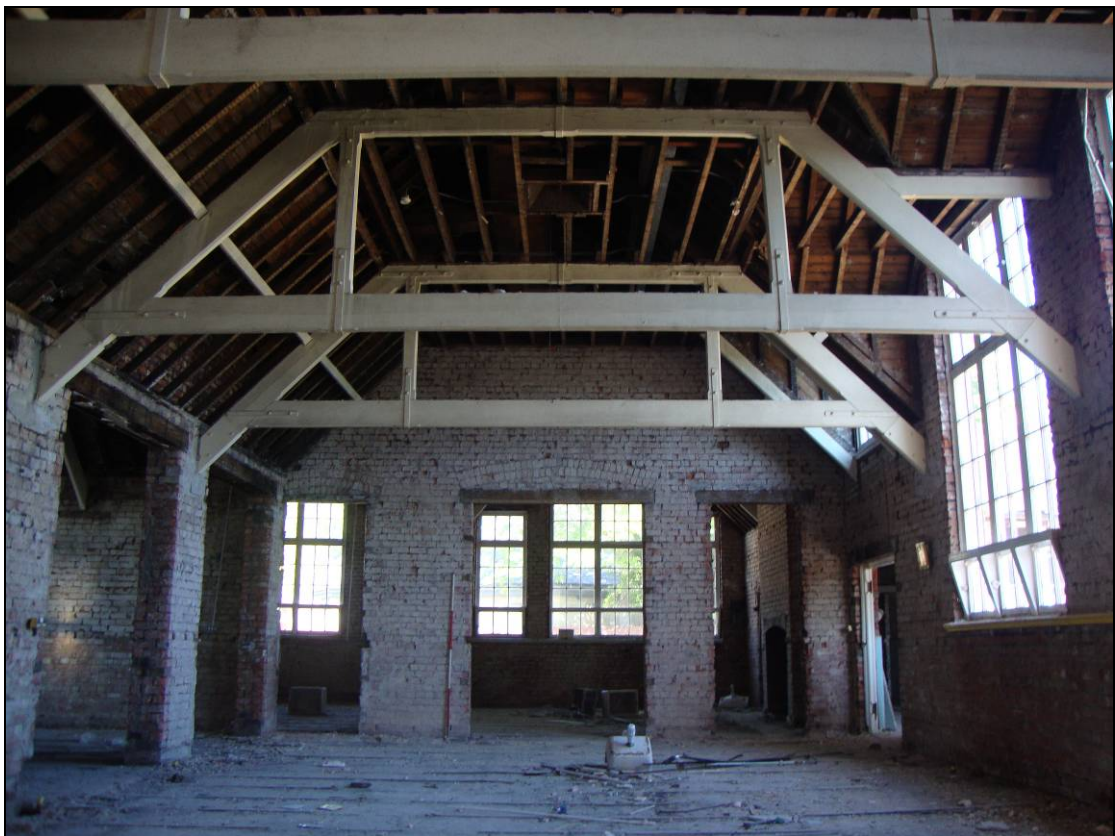
Figure 40: West elevation of Room 4, looking west. Scale = 2m
